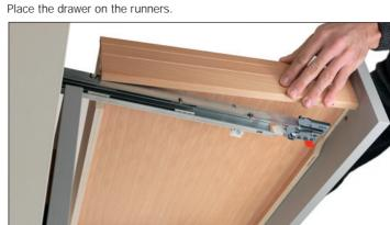
Close the drawer in order to locate it onto the locating pin of the runner.
